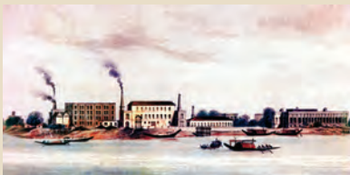
The Dhaka Sugar Company Works, popularly known as the Mill Barracks and the manager's residence.
