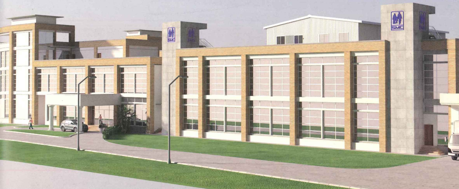
Model of 8 th to 12 th lines of production at ORS Factory, Bhaluka
