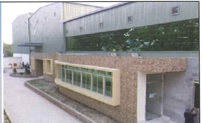
Partial construction of Health and Hygiene Factory in Comilla.
